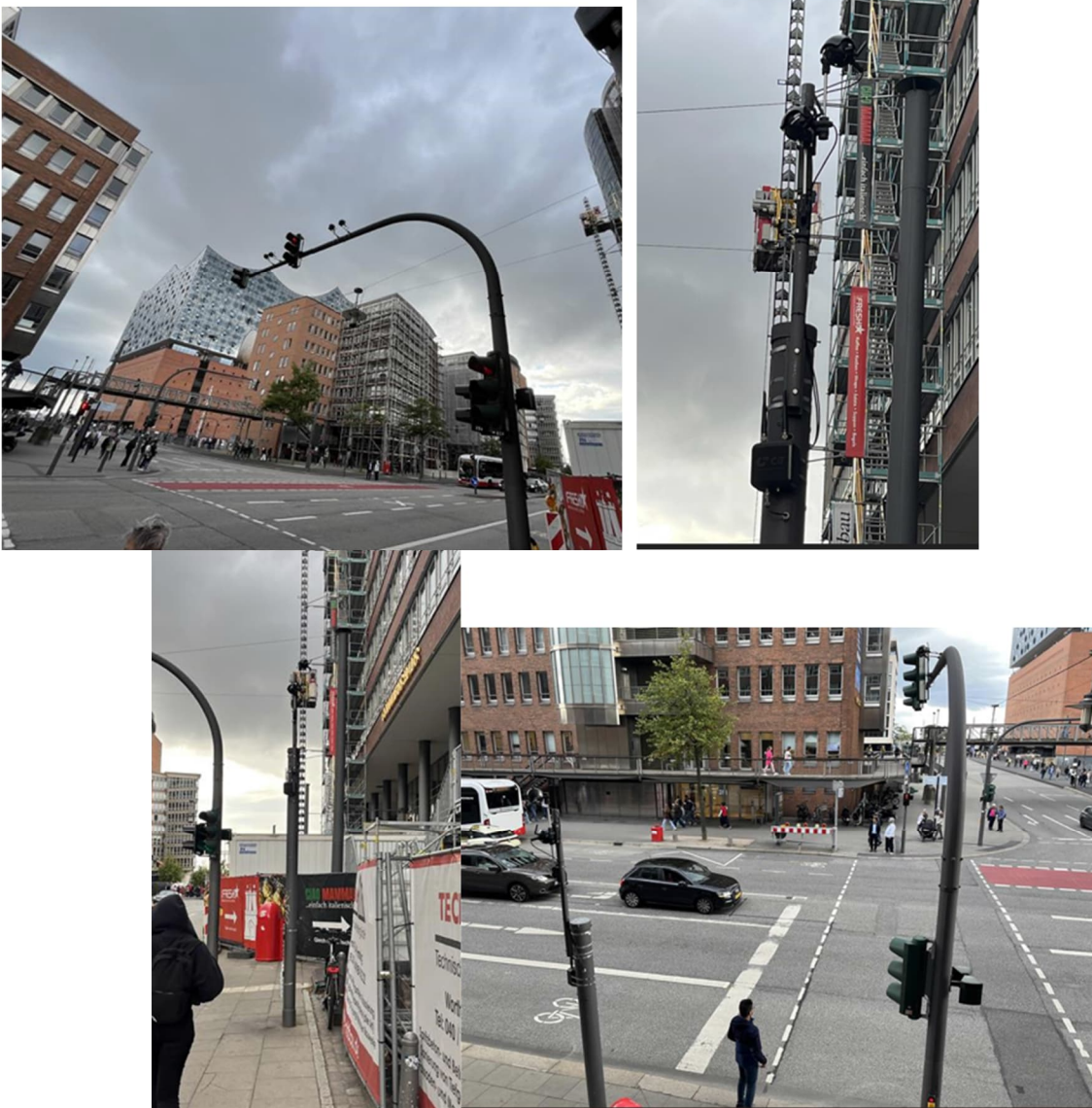
Figure 46 Pole used for equipment mount at P2-HH
